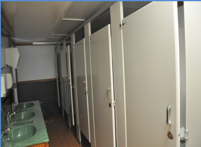
Hand wash area, women's stalls and urinals
